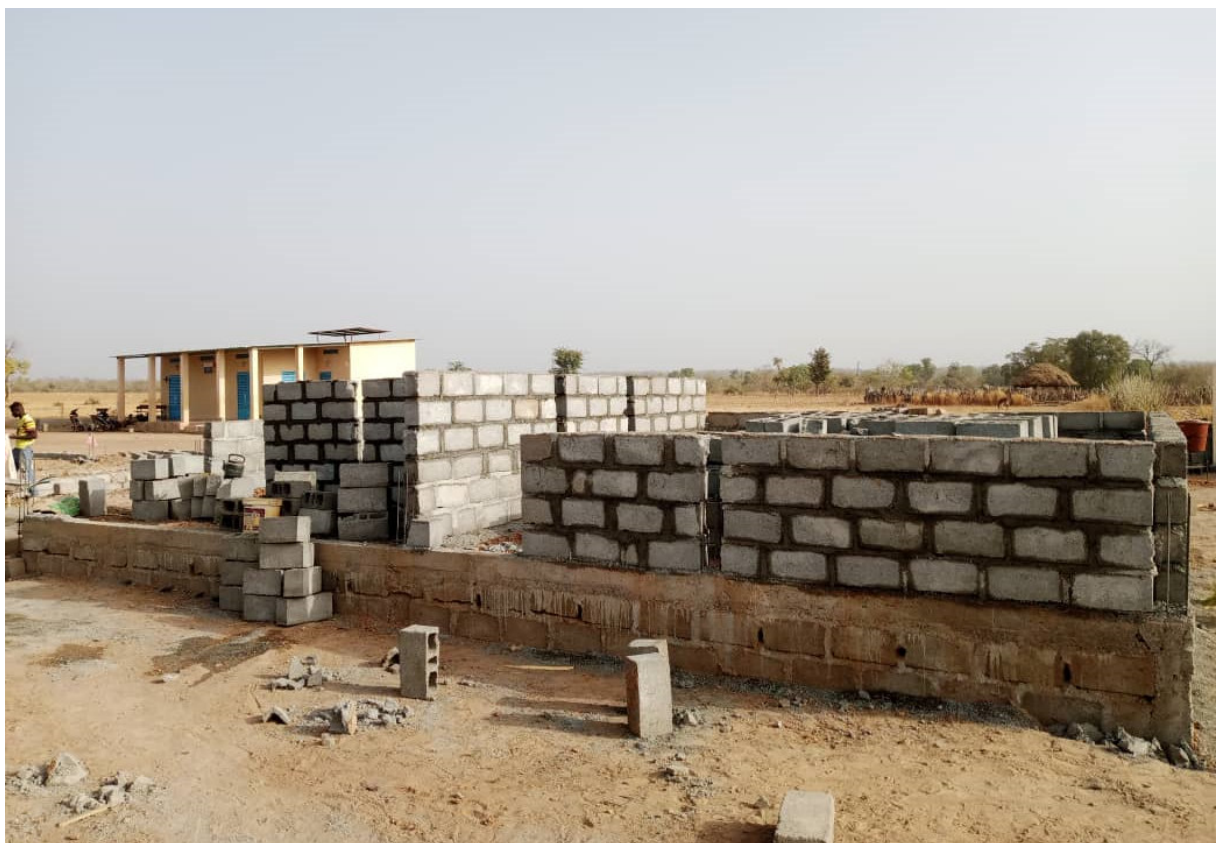
Perimeter walls under construction
