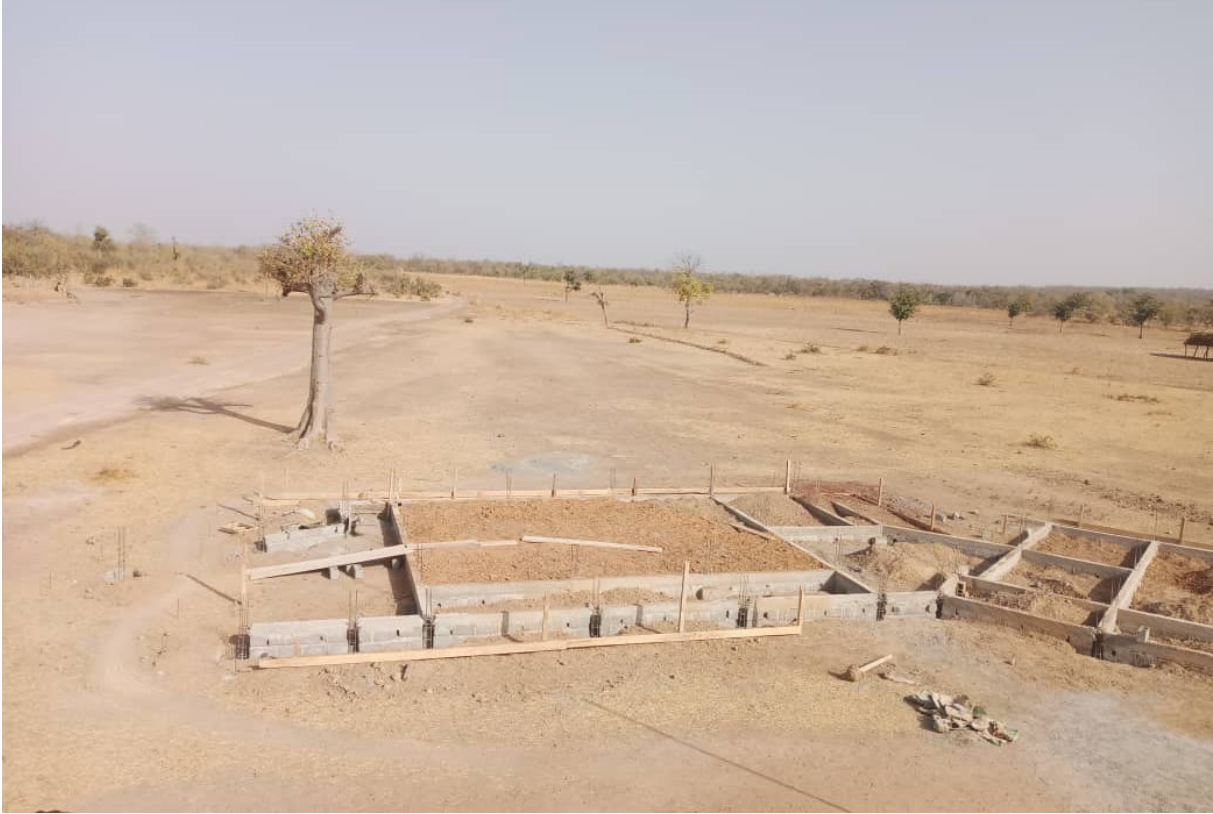
Third classroom, base ready
