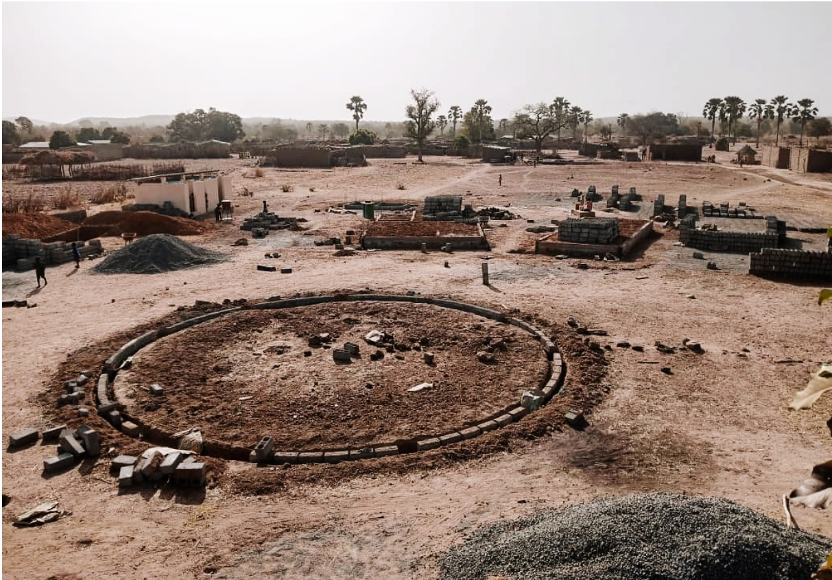
construction of the stage
