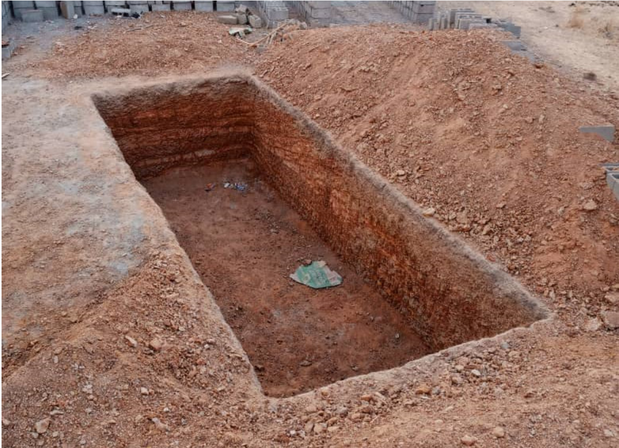
Pit excavation completed
