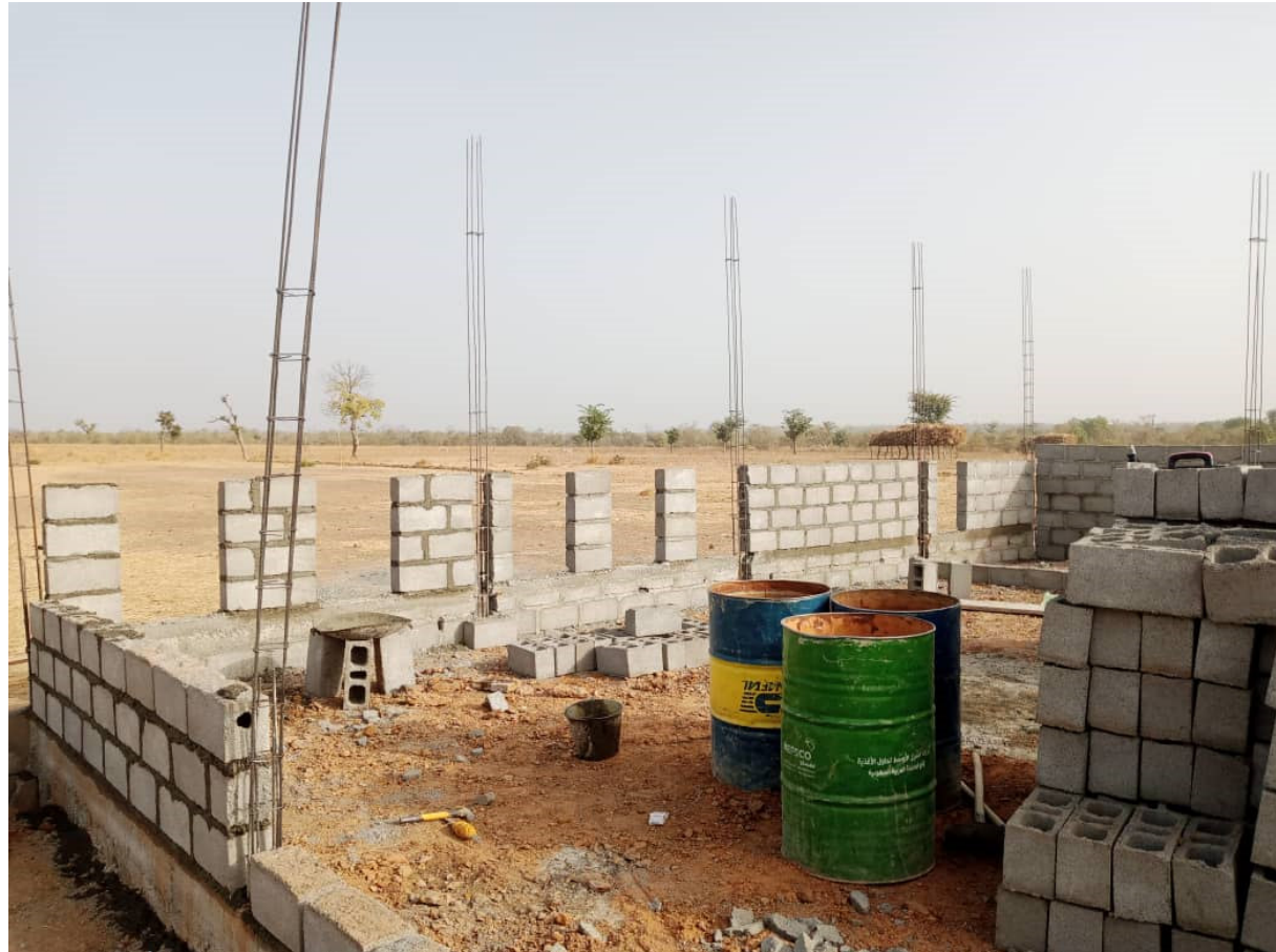
Perimeter walls under construction
