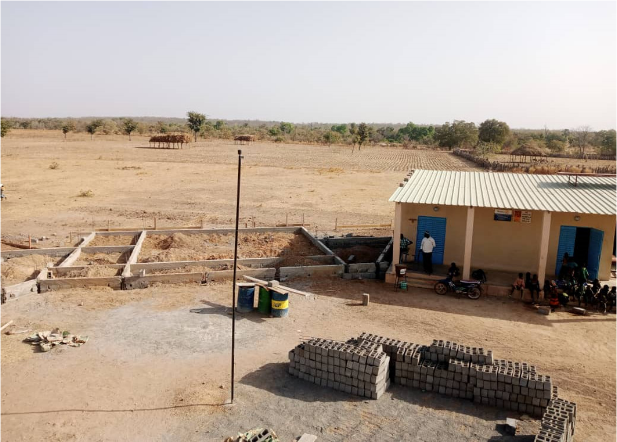
Second classroom, connected to the existing classroom. Base ready
