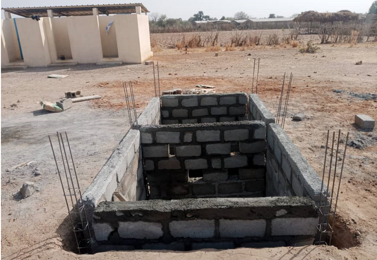
Perimeter walls under construction
