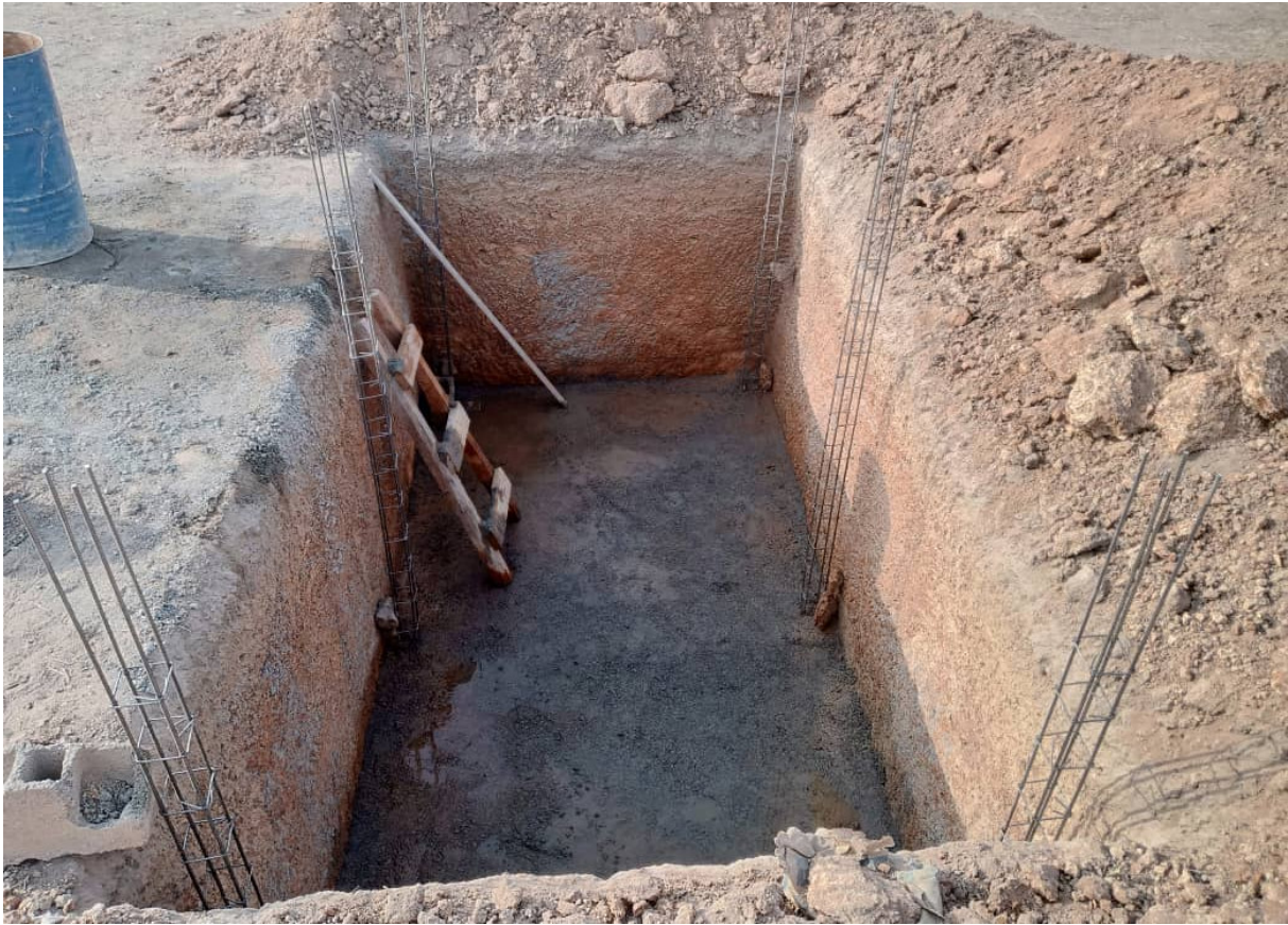
Pit excavation completed
