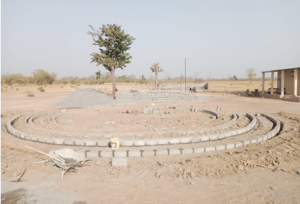
Construction of the seats
