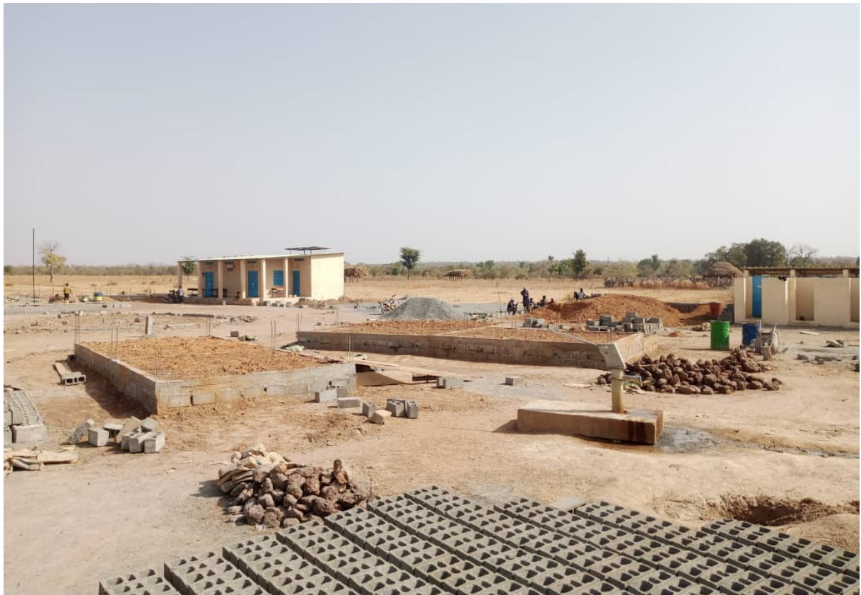
Base of the apartments ready
